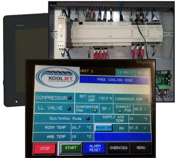
*KoolJet provides a comprehensive yet user-friendly interface to the control system settings. The "Master" and all "slave" units are accessible from one screen that is connected using common control wires. Each KoolJet slave can have its own temperature and humidity settings. This strategy maximizes the ability to store some produce for short term and some for long term.*
